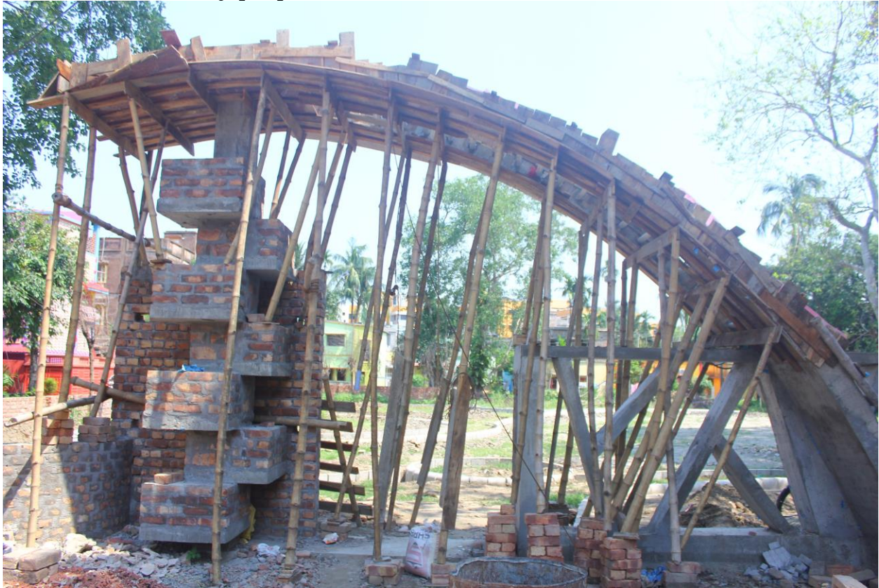
Park under Renovation at Ward No. 33
