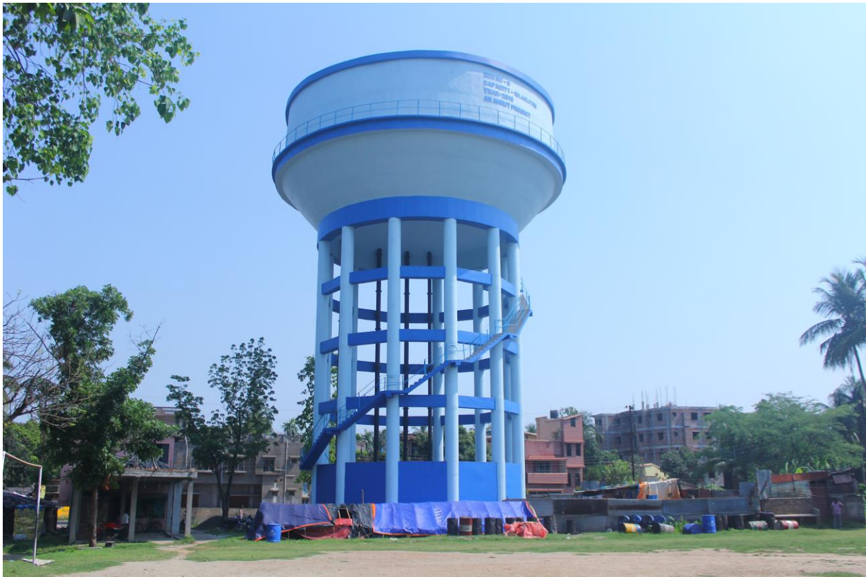
Elevated Service Reservoir at Ward No. 34
