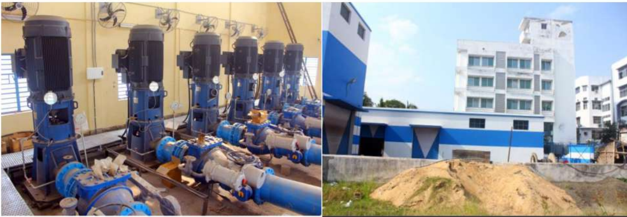
Under Ground Reservoir at Ward No. 08
