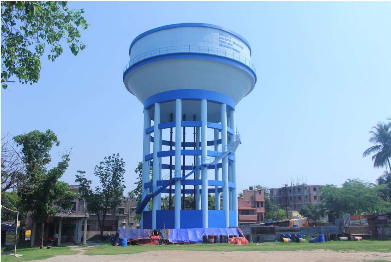
Elevated Service Reservoir at Ward No. 34
